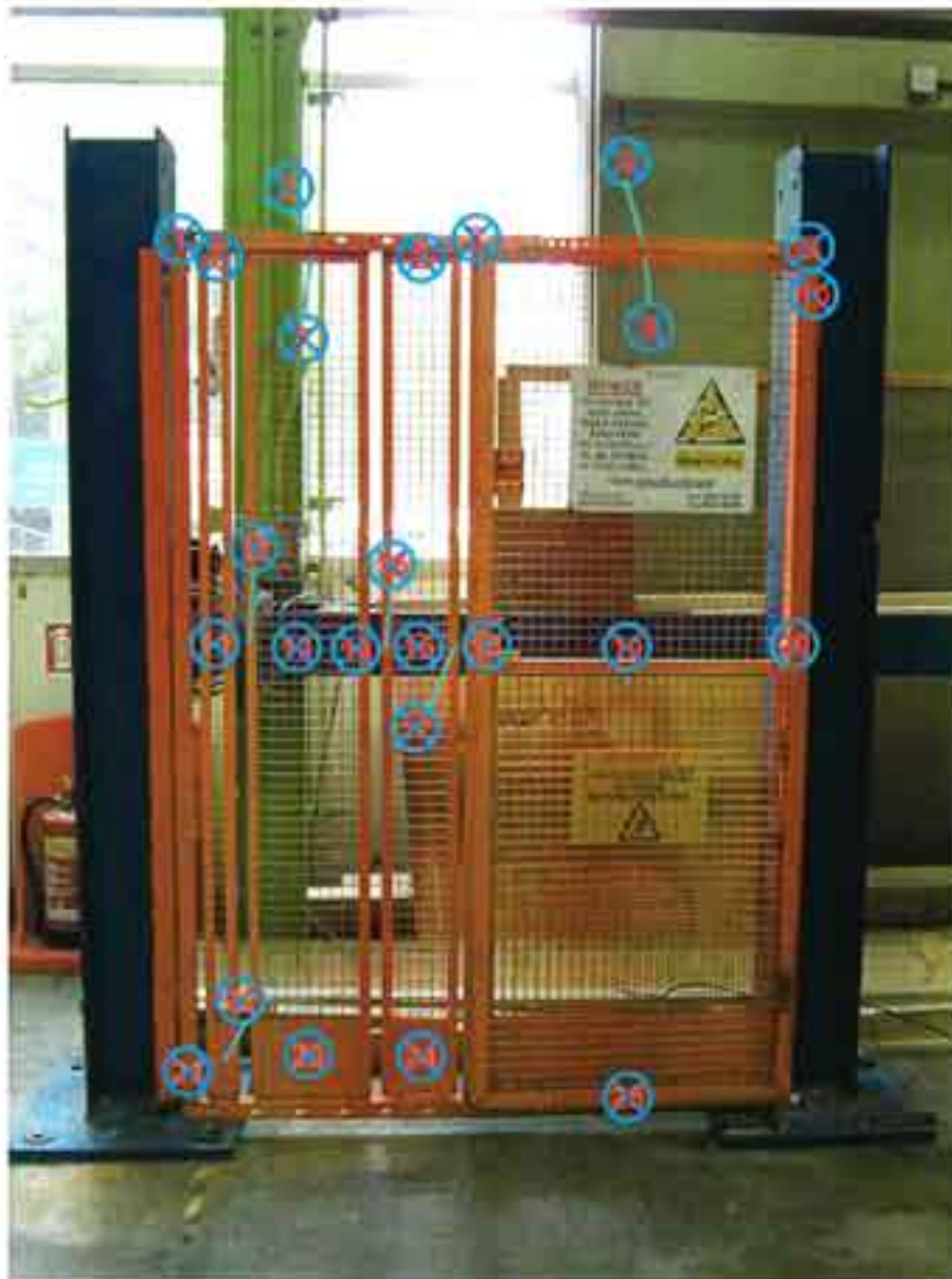
Figure A3: Horizontal static load test locations with main door open.
