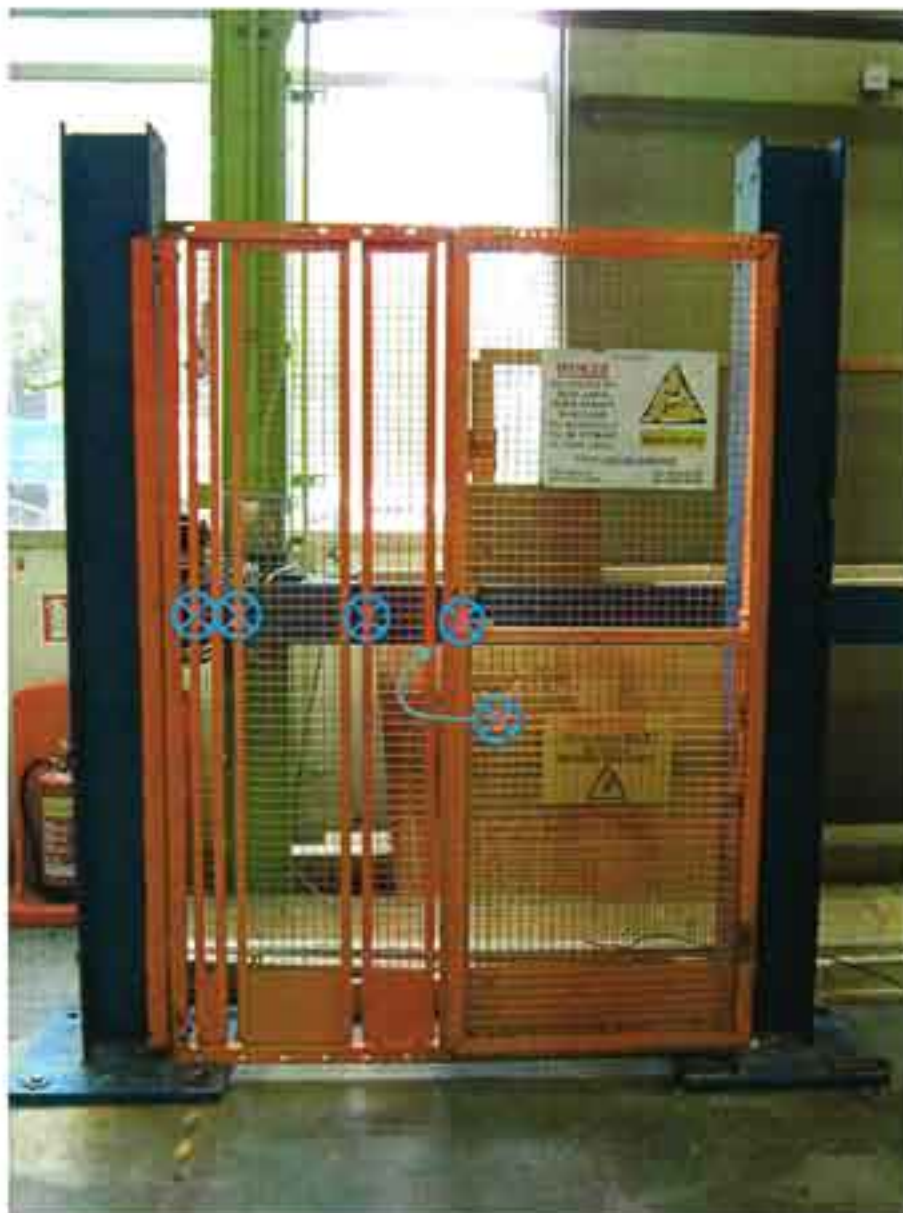
Figure A5: Parallel static load test locations
