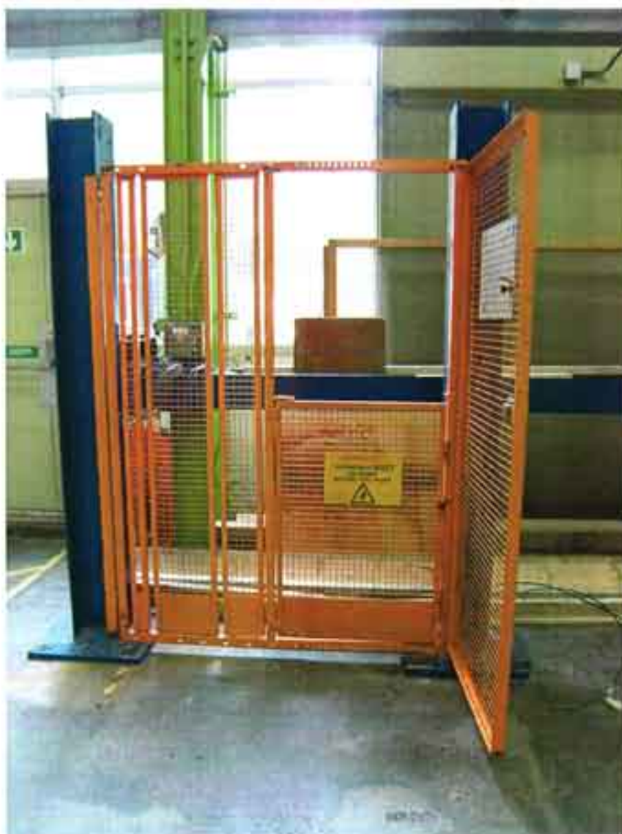
Figure A2: Fullgate lift shaft safety gate system with main door ajar
